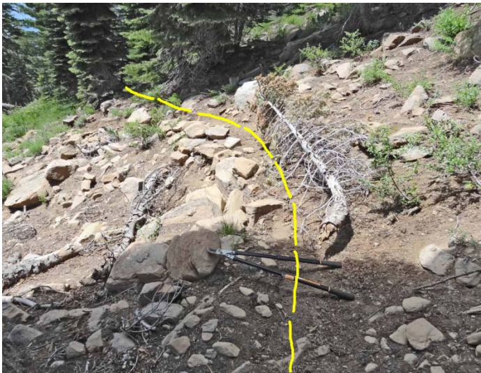
At Left: The heavy winter snows have deposited a short dead tree into the trail-bed. At Right: the tree is side-cast on the downhill slope where gravity and future winter storms will take it even further away from the trail-bed. This appears simple enough; yet previously, no wilderness hiker had paused to do this simple task. The cogent insight is: side-cast of fallen dead trees only takes one minute with no tools required, and it is important for the safety of our Tevis horses inside the Granite Chief Wilderness Area within Tahoe National Forest.
